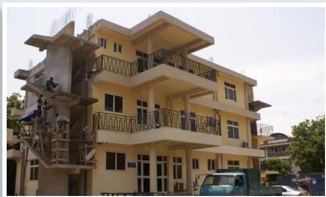
New UGMS Research Building Complex (1 st Floor)
